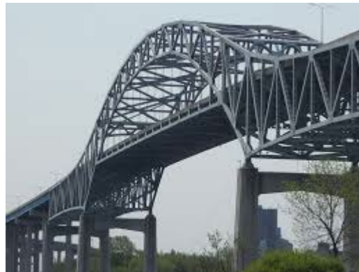
Structural health monitoring (Large area strain sensors)
